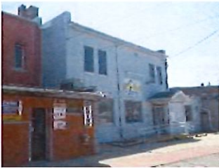
Top: During construction Bottom: Before renovation
