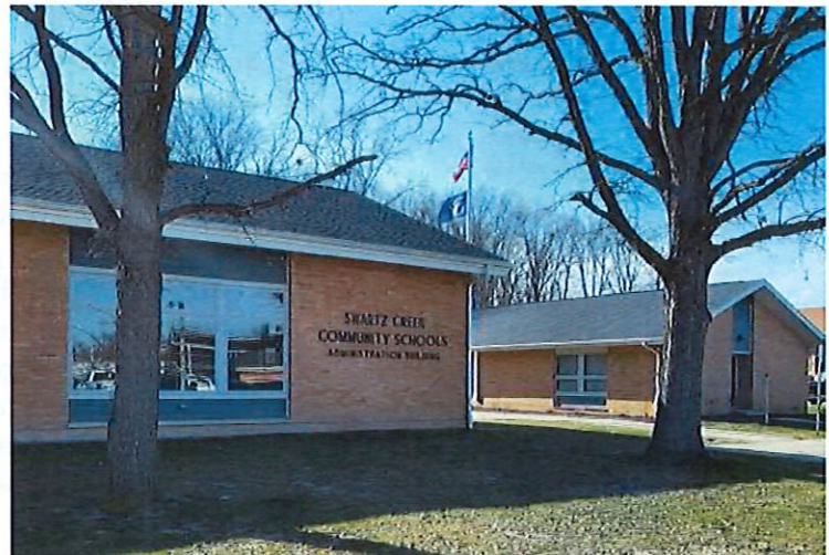
Board Room addition, left side. Original building, right side
